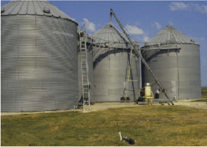
Well maintained storage facilities & surroundings
